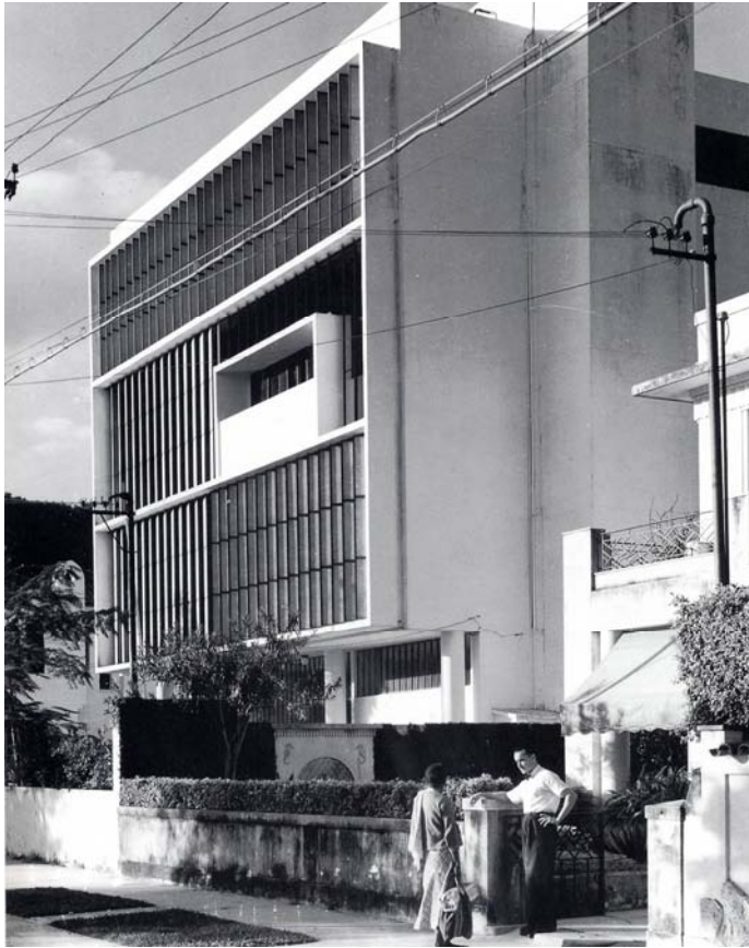
The Obra do Berco in Rio de Janeiro demonstrates Niemeyer's commitment to finding solutions to buildings erected in a tropical environment. He introduced adjustable vertical louvres (brise-soleil) to the building to control the heat from the tropical sun
